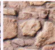
Wide Mortar Joints, Raked
