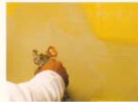
Sto EmeraldCoat is specially formulated for use under stucco and other claddings
